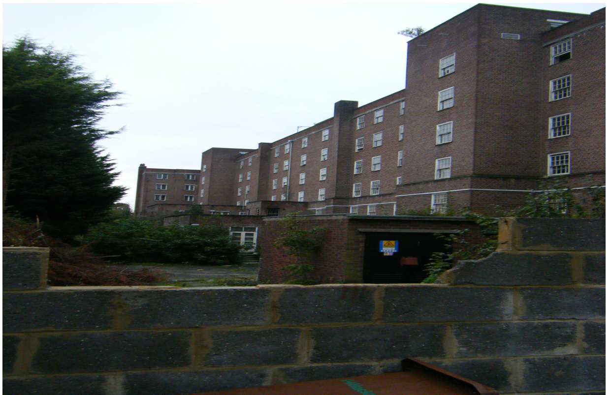
Rear of Buccleuch House
