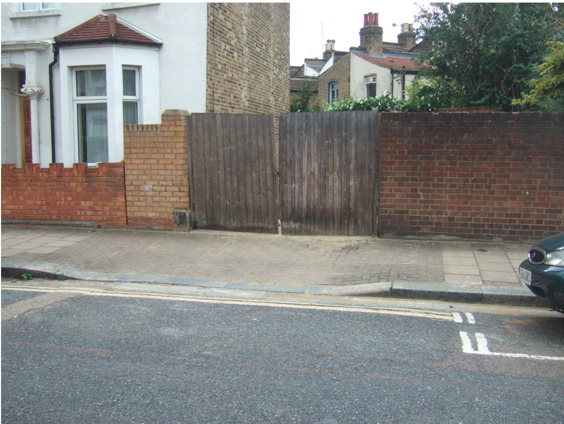
Figure 2: Looking west from Aden Grove at 58 Aden Grove and proposed area of development
